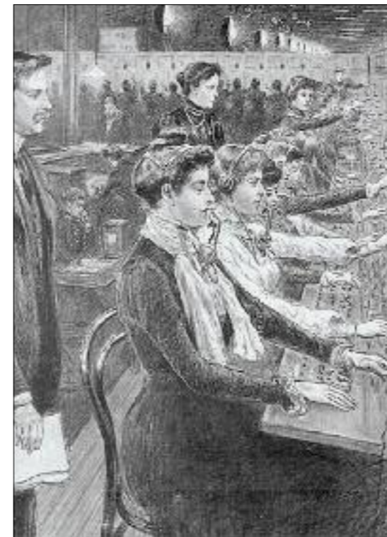
A telephone exchange in 1902. In early exchanges, only callers attached to the same exchange could be automatically connected. Long-distance calls between cities and countries required three or four operators to connect them.
